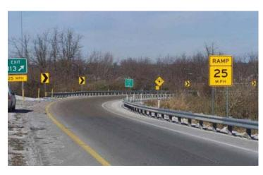
challenging curves, dual indicated advanced signs with constant flashing beacons may be effective. Pavement markings are also an effective communication tool to indicate the alignment change. Pavement friction is critical for changing vehicle direction and ensuring the vehicle remains in its lane. Traditional friction courses or high friction surface treatments should be considered for curves with numerous wet weather crashes or severe curves with higher operating speeds.
