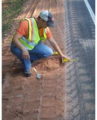
somewhat effective in mitigating the severity of crashes involving pavement edge drop-offs. However, constructing a durable edge was not perfected until the 1990s, and during development it was found that a flatter, 30 degree angle was easier to construct. Additional testing indicated that the 30 degree edge improved the chances of a safe recovery.
