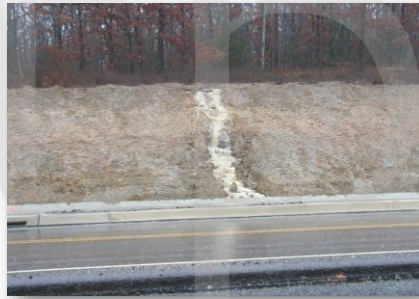
Gully Erosion (concentrated flow)
