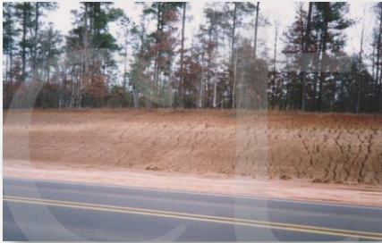
Rill Erosion (small, defined flow channels)
