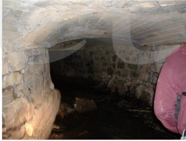
Tunnel at Park Ave.
